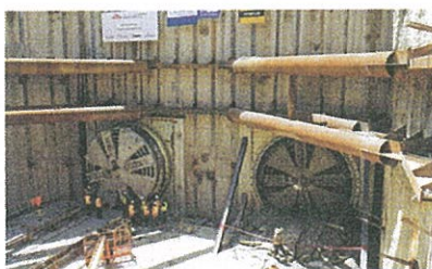
Jobsite at Toronto-York Spadina Subway Extension
